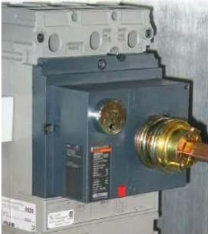
Figure 2-2: Lockout/Tagout (MTD0525)
